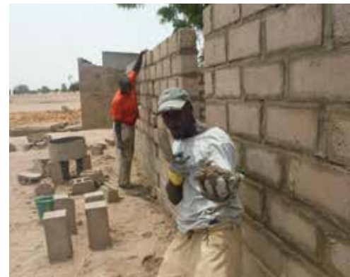
Community volunteers building walls for teacher housing adjacent to the school.
