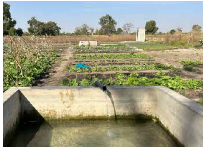
Something as small as upgrading old valves helps prolong the life of infrastructure and conserve vital water resources.
