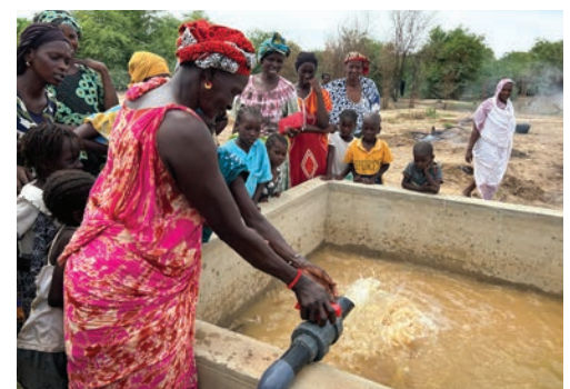
Garden President Fatimata Sekk verifies that all infrastructure is completed and functioning properly. This garden draws water from the river, which turns brown with silt after it rains.
