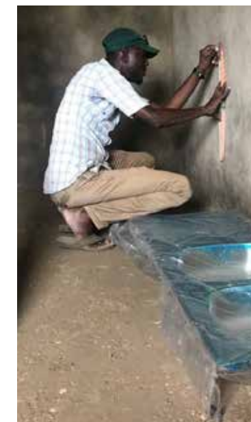
Installing plumbing and sinks at Keur Ngor health post.
